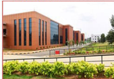
Bangalore, India –Receiving plant
