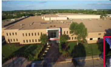
Lincoln, Nebraska Sending Plant
