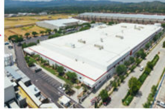
Nogales, Mexico Receiving Plant
