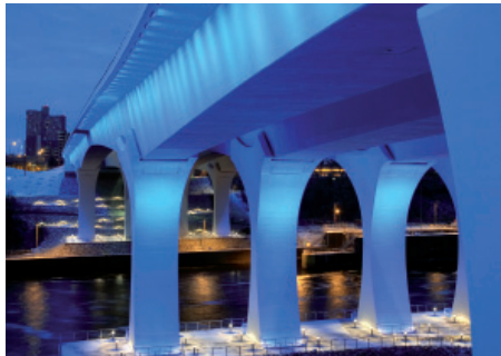
Bridge / Road Infrastructure lighting
