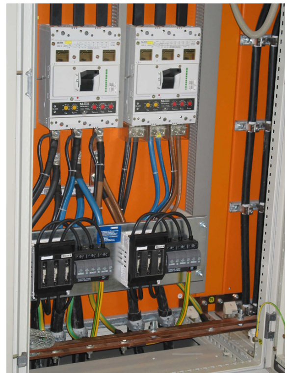
Figure 11 100 kA SPD for use at power line input feeds
