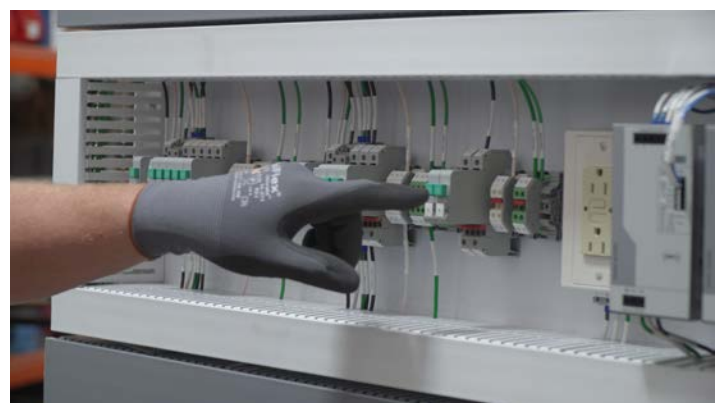
Figure 4: Circuit breakers protect the AC equipment within the panel.
