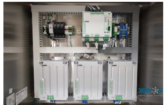
Figure 1: The AC UPS system, based on the 500 VA QUINT AC UPS.
