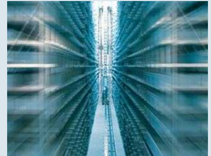
Wireless LAN in high-bay warehouse systems
