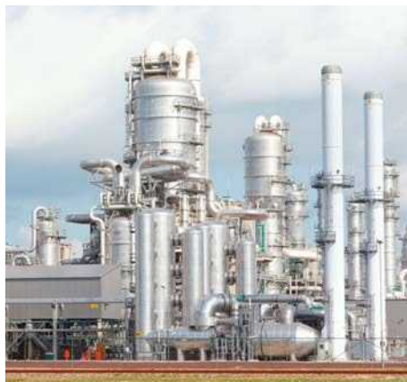
System expansion and post installation
