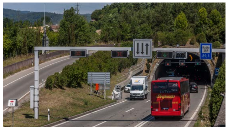
Fig. 3 The sign gantry at the entrance to the Cholfirst tunnel is equipped with a dynamic traffic control system.
