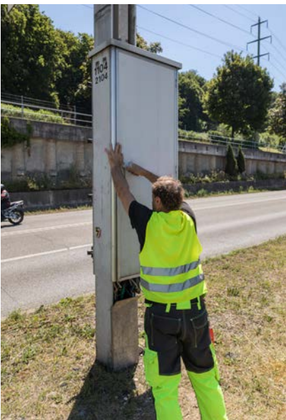
Fig. 5 The control boxes installed in the tunnel entrance zone are difficult to access.
