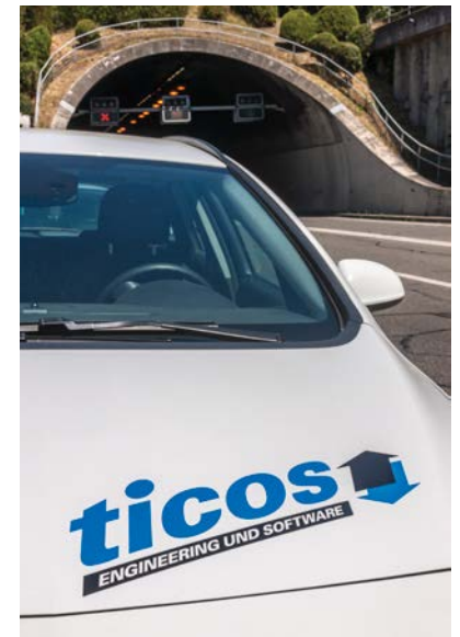
Fig. 1 Ticos Engineering & Software AG specializes in tunnel and traffic control technology.
