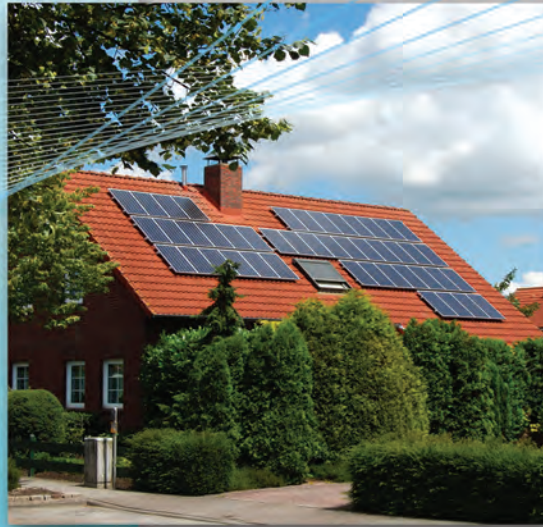
Energy Generation - Solar PV Systems
