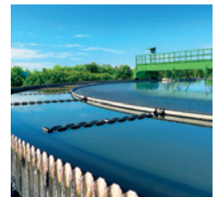
Waste Water Treatment
