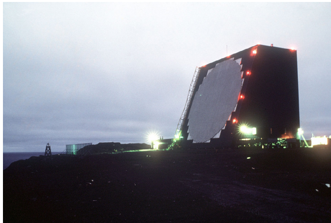
Figure 2. The COBRA DANE radar is a single faced ground-based, L-band phased-array radar located in northern U.S. Indo-Pacific Command (USINDOPACOM) area of operations and operated by the U.S. Air Force. Source.
